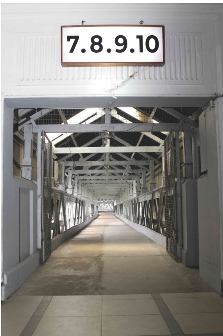
One of the two bridges leading to the train platforms located at a lower level.
