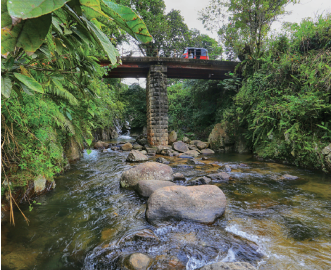
A trail past the Kota Ganga bridge leads to the cool water downstream.
