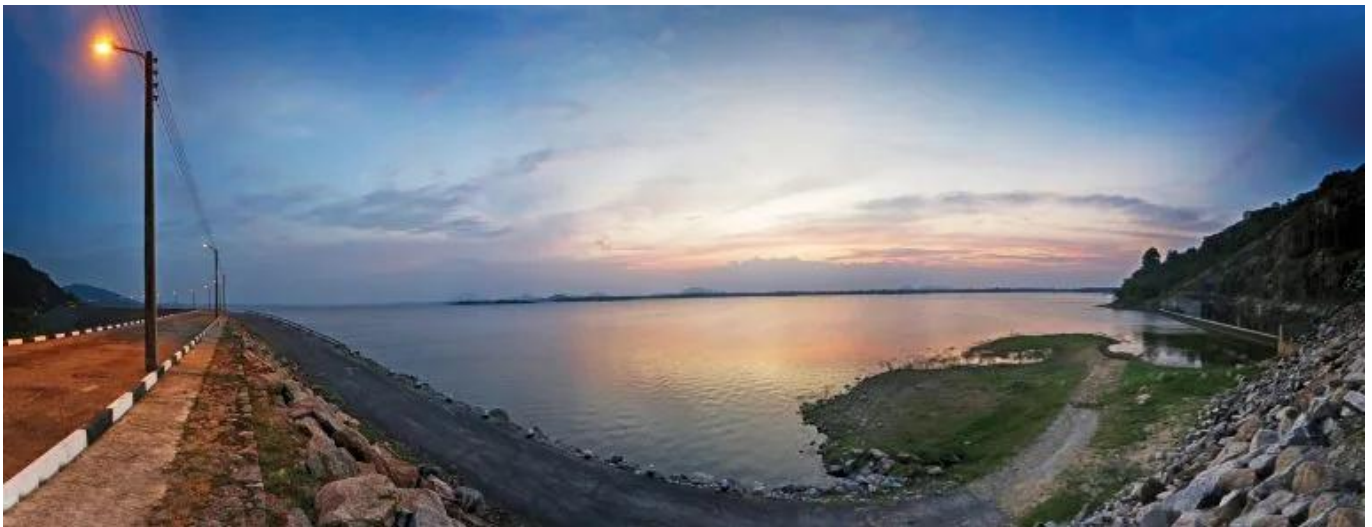
The vast Maduru Oya Dam is situated 40km South of Manampitiya.
