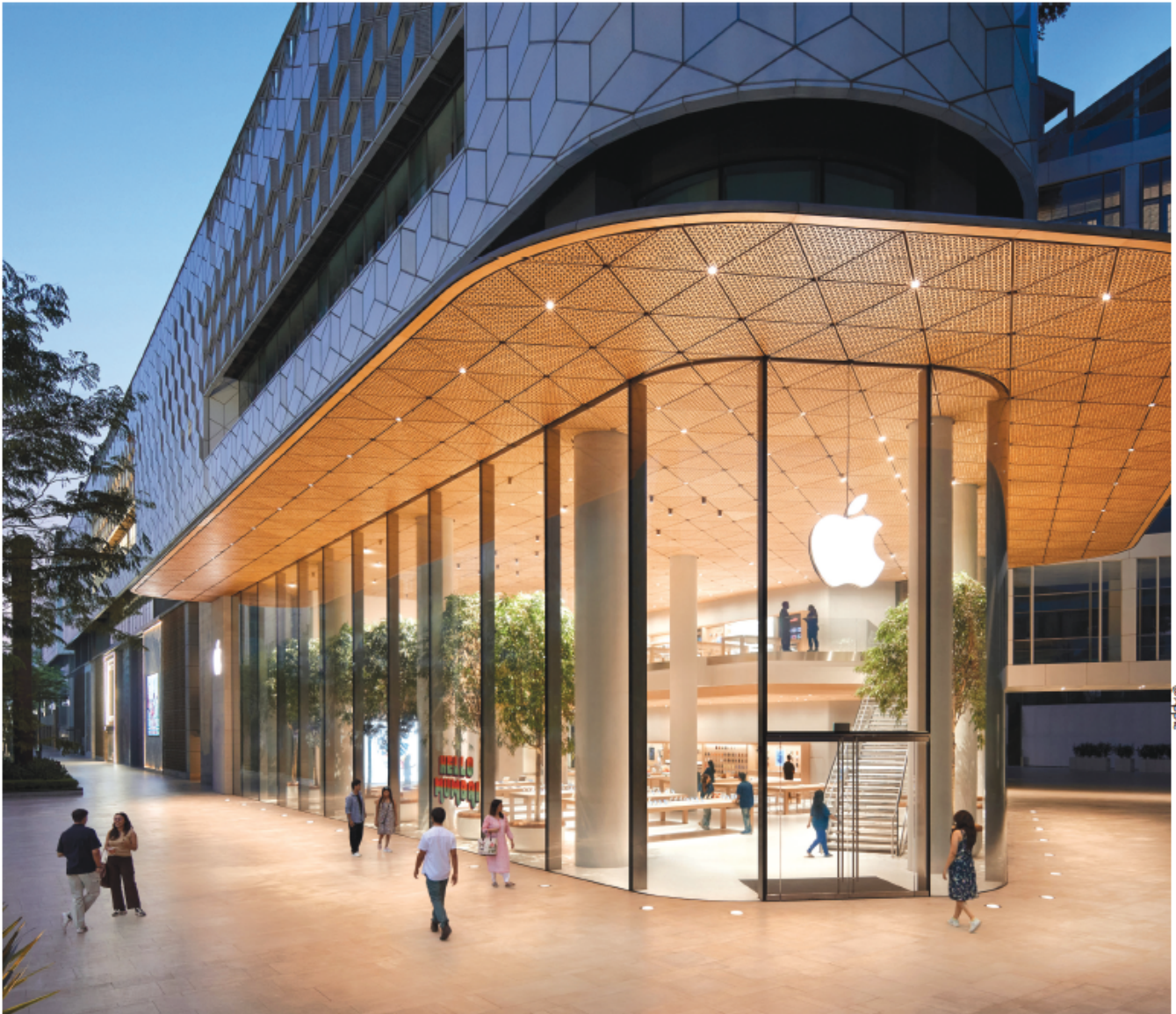
Apple BKC at night. The 8-meter-tall glass façade enhances this seamless connection between the generous double-height volume and the outdoor areas. A row of ficus trees, along the inside of the glazing, accentuates the store's relationship with its landscaped surroundings.
