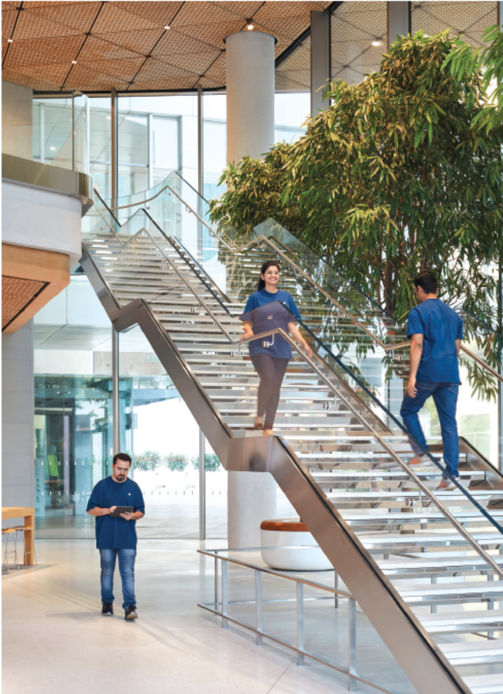
Detail of staircase to mezzanine. A striking staircase, made of stainless steel and two 14-meter-long glass balustrades, creates a delicate connection between the ground level and the cantilevered mezzanine.
