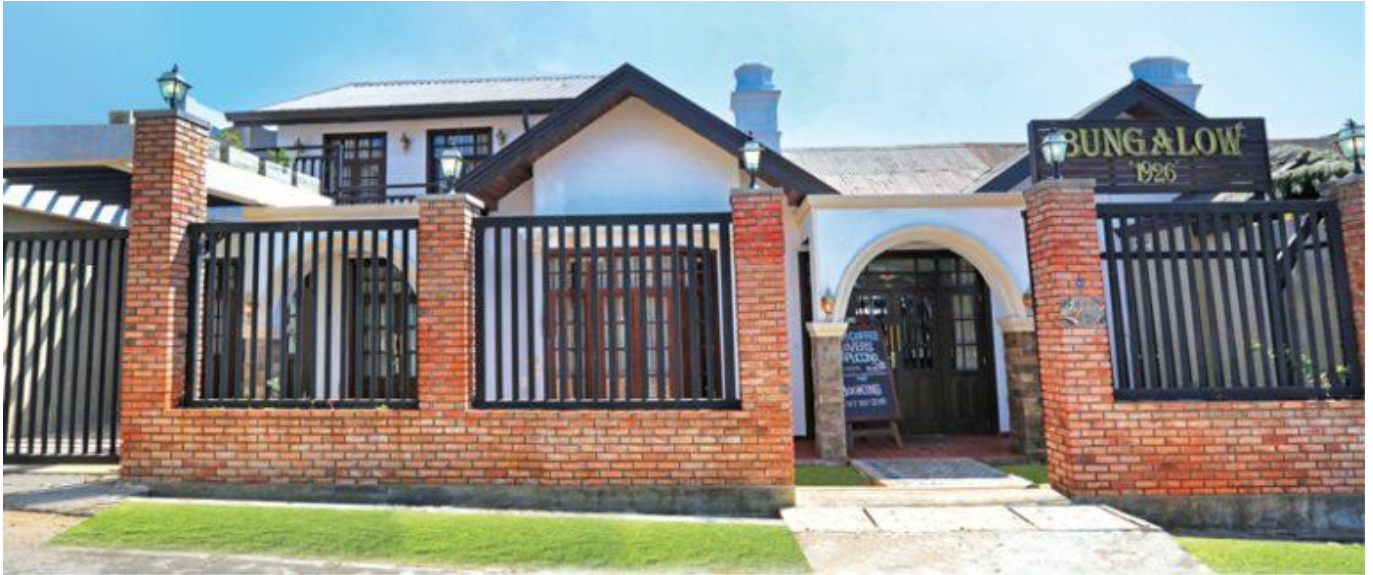
The colonial façade of Bungalow 1926
