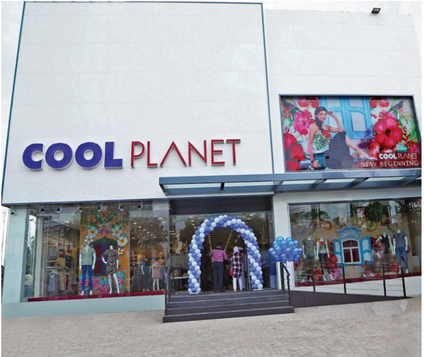
Façade of Cool Planet Maharagama
