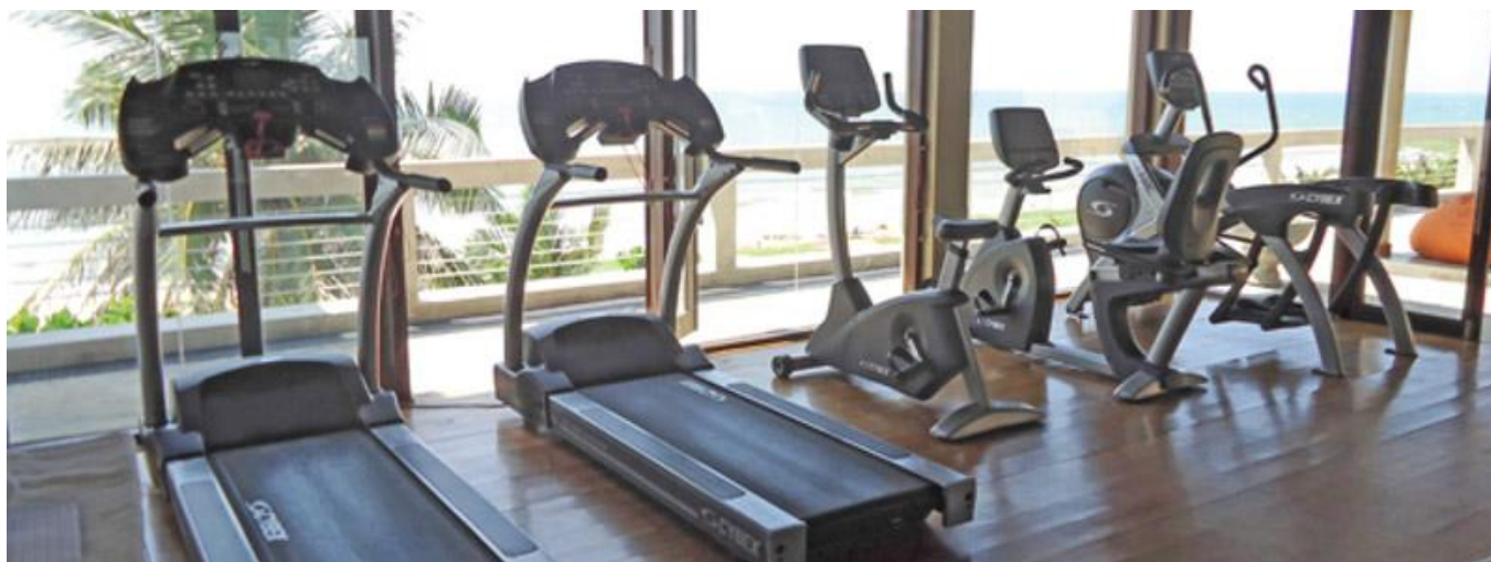
Pro3 Treadmill, 750AT Total Body Arc CrossTrainer, 750C Upright Bike, 750R Recumbent Bike, The rooftop gym at Jetwing Sea, Negombo
