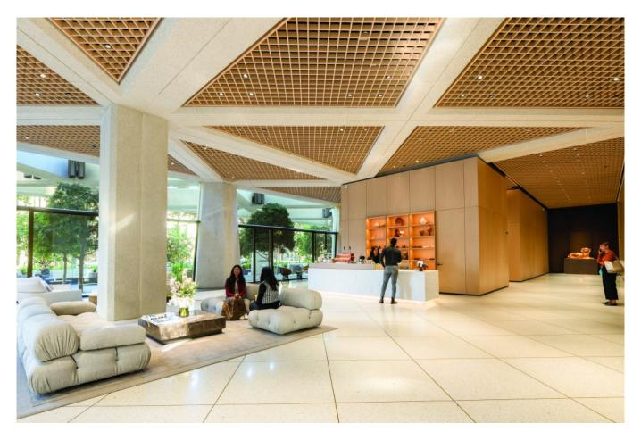
The tower's lobby has been redesigned to emphasize the building's powerful structural rhythm. A forensic study of the original building blueprints showed a spectacular diagonal structure, which was hidden above the ceiling. This structure has been revealed and clad to match the building's exterior, creating a seamless transition between inside and outside.
