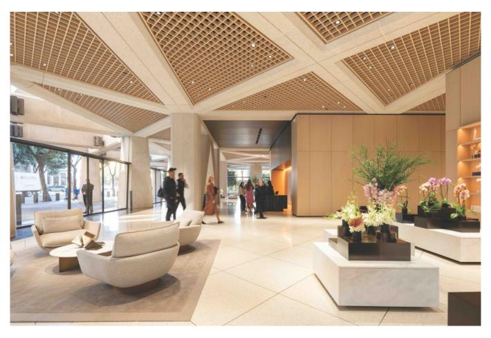
The tower's lobby has been redesigned to emphasize the building's powerful structural rhythm. A forensic study of the original building blueprints showed a spectacular diagonal structure, which was hidden above the ceiling. This structure has been revealed and clad to match the building's exterior, creating a seamless transition between inside and outside.
