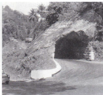
Kadugannawa Pass — cut through the rock. A constant reminder of British Engineering skills. (Suresh de Silva).
