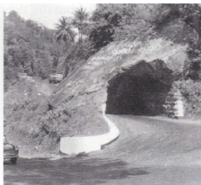
Kadugannawa Pass — cut through the rock. A constant reminder of British Engineering skills. (Suresh de Silva).
