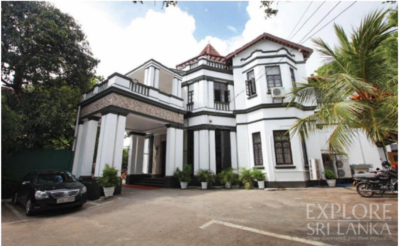
The exterior of Peach Valley
