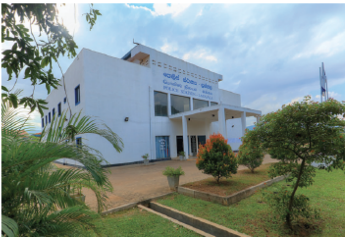
The Police Station is an eco-friendly space.
