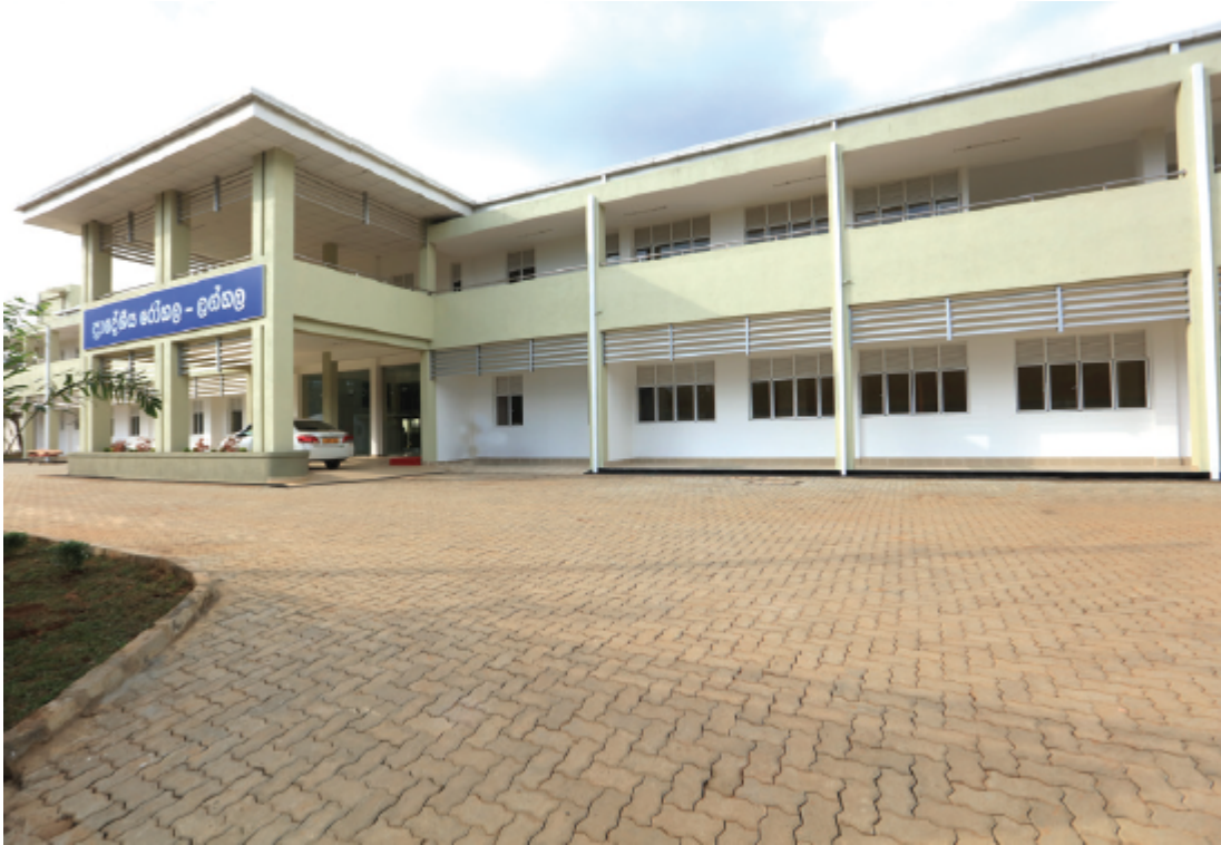
The Divisional Hospital is fully functional despite being established recently.
