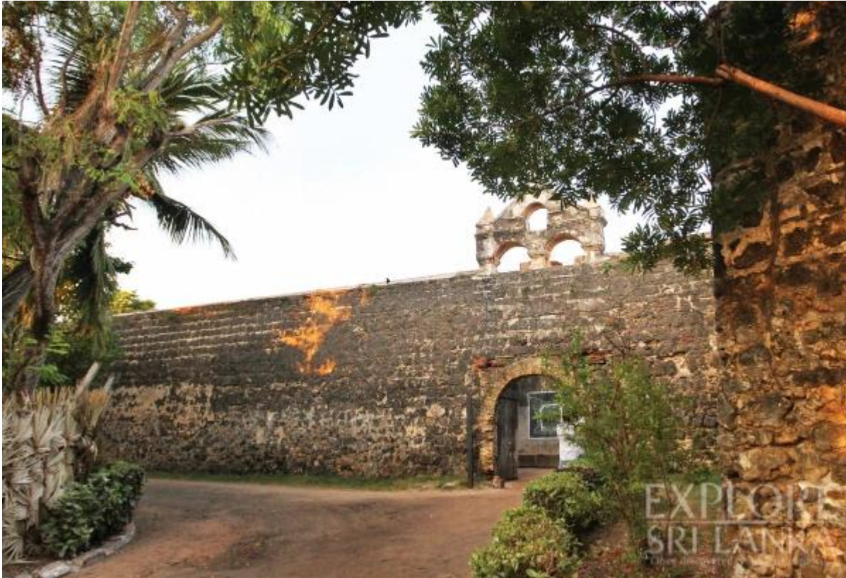
The single entrance to the Kalpitiya Fort
