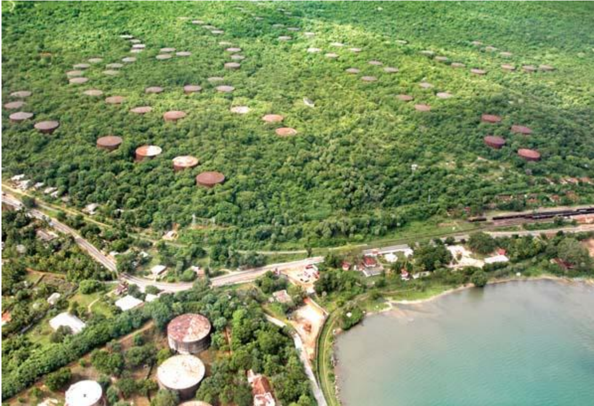
The aerial view of the oil tanks scattered around the land
