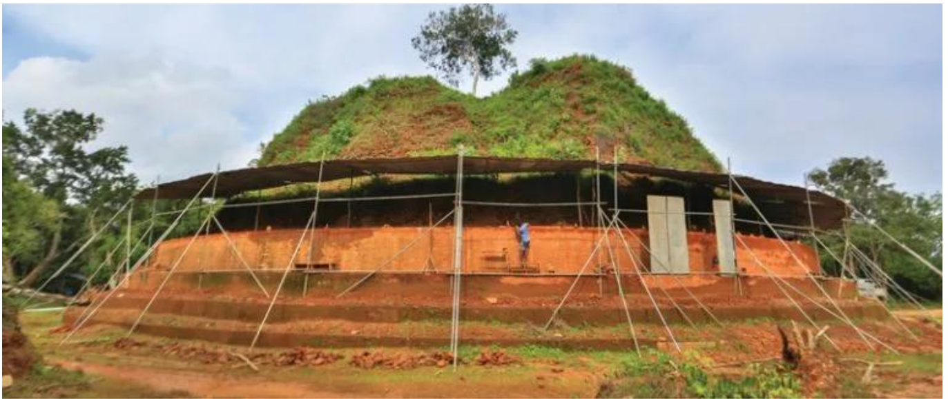
Neelagiri Maha Seya is being restored back to its bygone splendour
