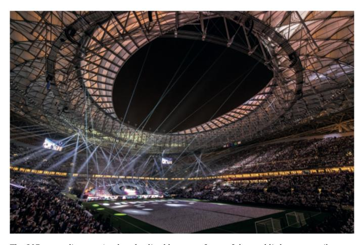
The 307-metre-diameter 'spoke-wheel' cable net roof, one of the world's largest tensile cable-net roof in a stadium.
