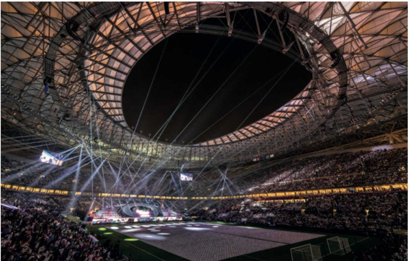
The 307-metre-diameter ‘spoke-wheel’ cable net roof, one of the world’s largest
