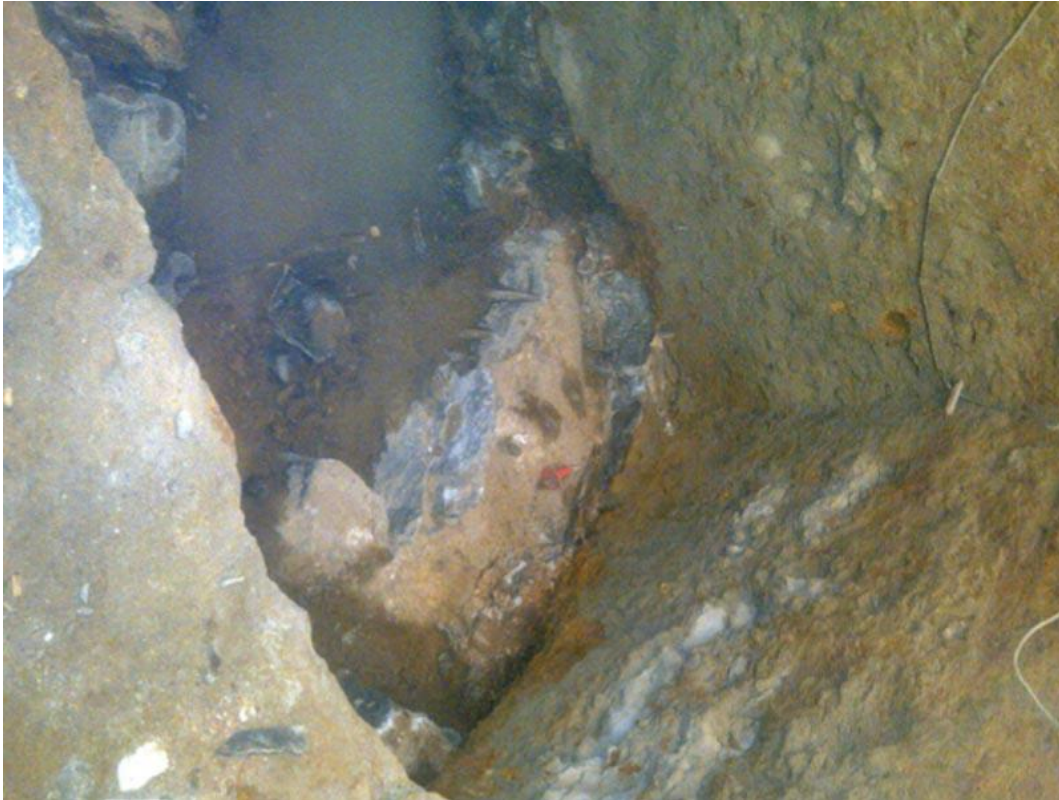
Part of the rock that surfaced while constructing the elevator shaft
