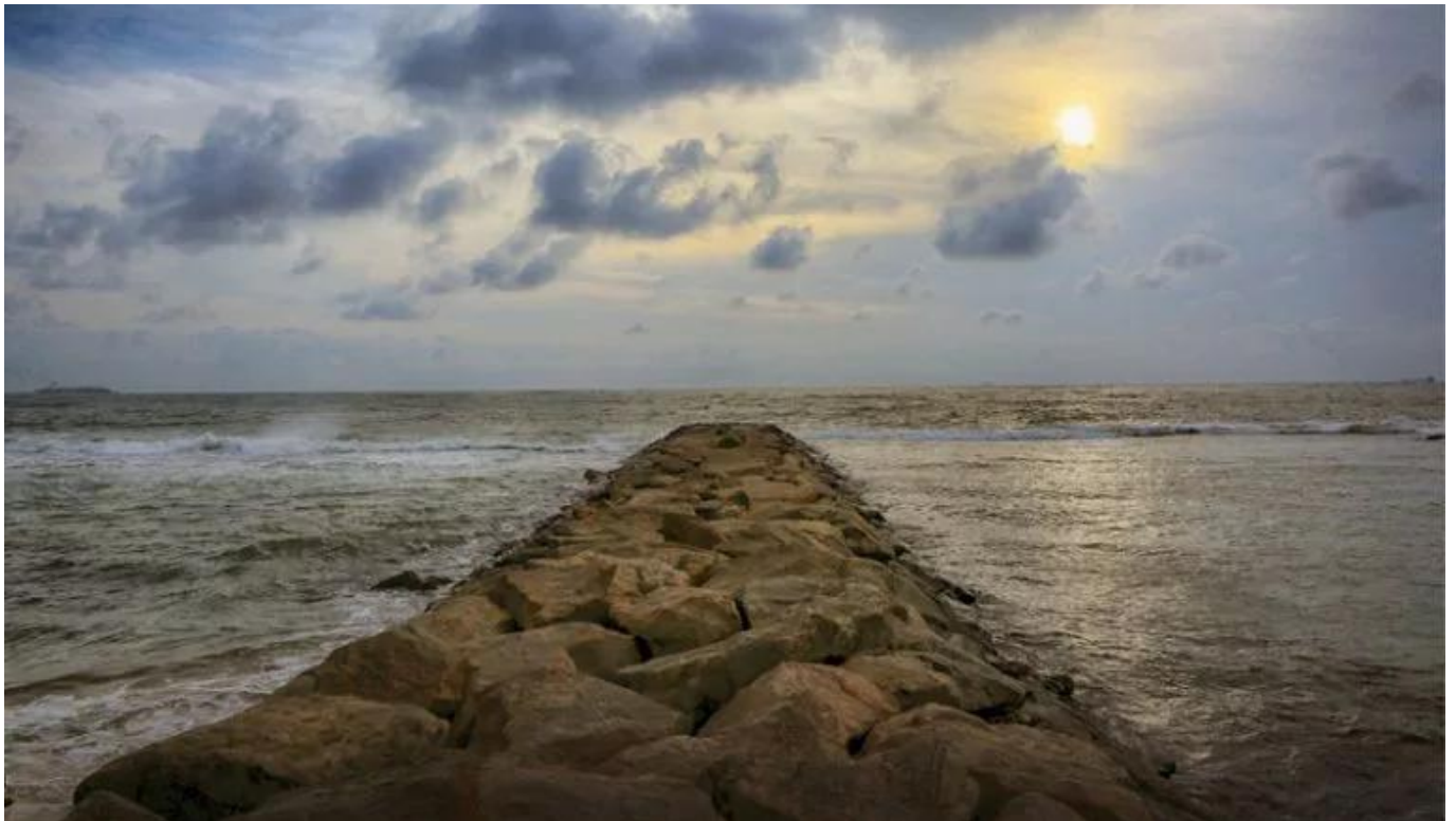
A breakwater stretches out to the sea
