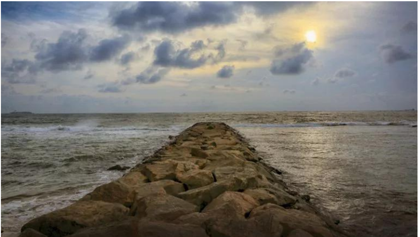
A breakwater stretches out to the sea
