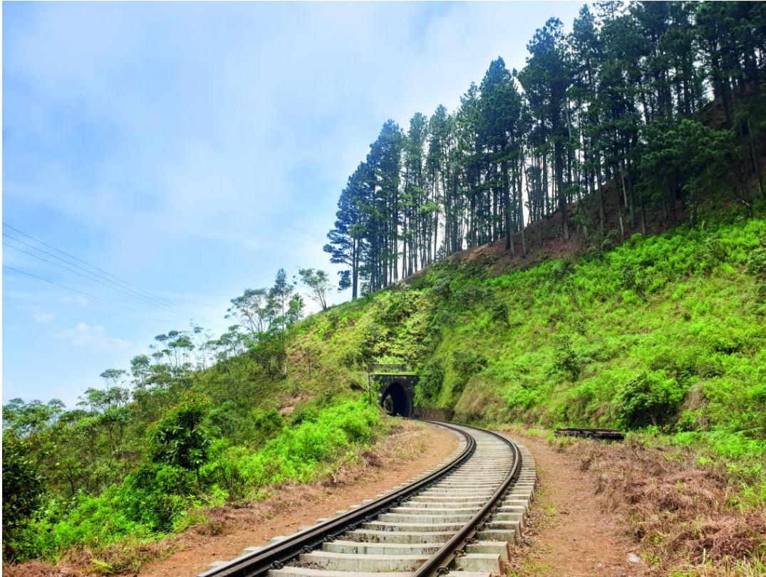
Tunnel 36 - a memorable feature in stage 12 is walking through a railway tunnel, the only such instance on the Pekoe Trail.
