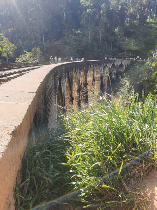
A closer view of the Nine Arches Bridge.
