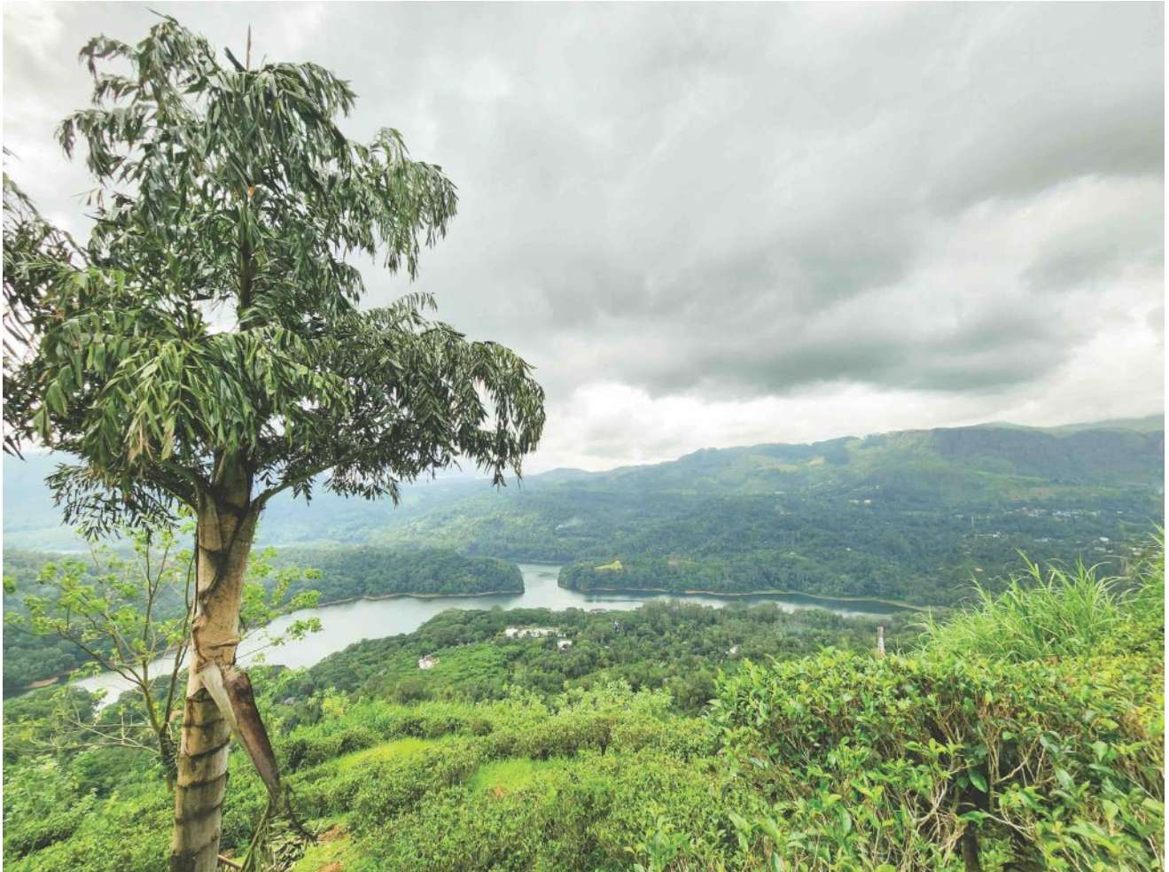
View of Kotmale Reservoir in stage four.
