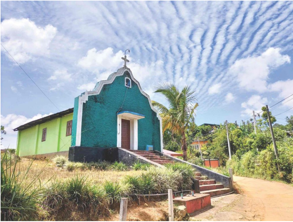
Thiruvallular Church in Darawala.
