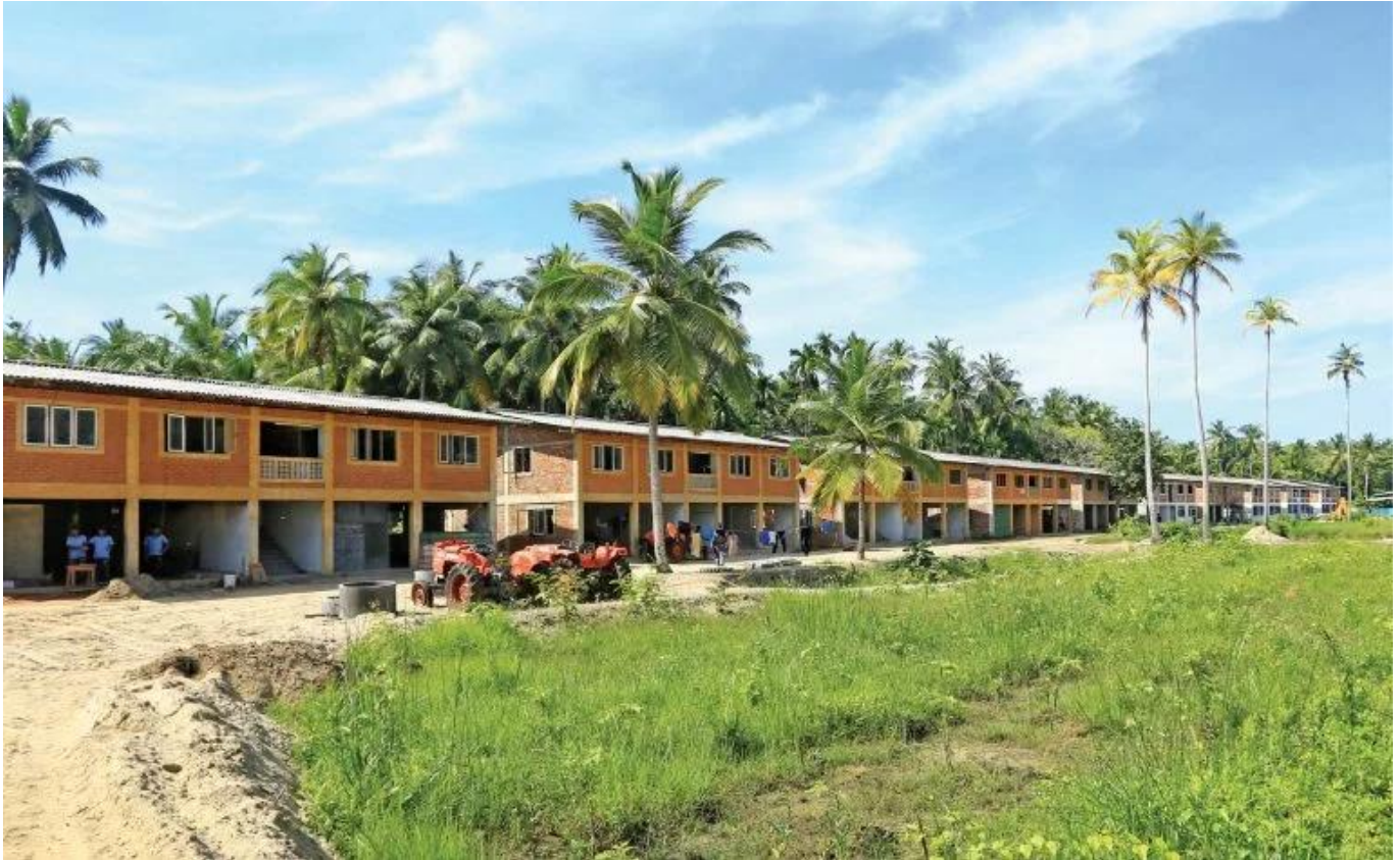
The complex of shop-house units at Seenigama
