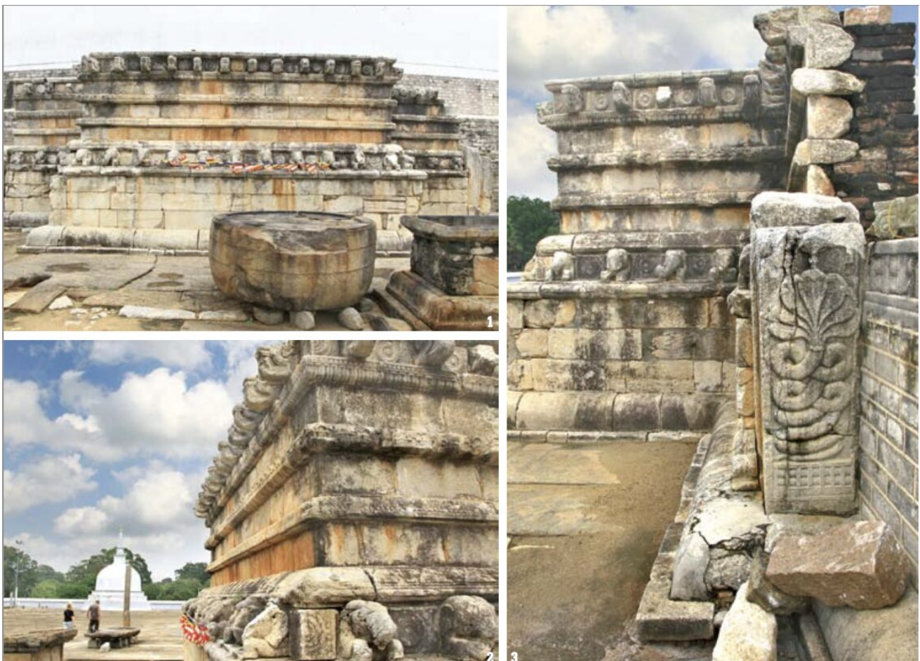
1. The ancient stone stages on which the flowers are offered to the Stupa 2. Traces of the paintings are still visible on the Wahalkada 3. Ruins of the ancient Wahalkada on the West
