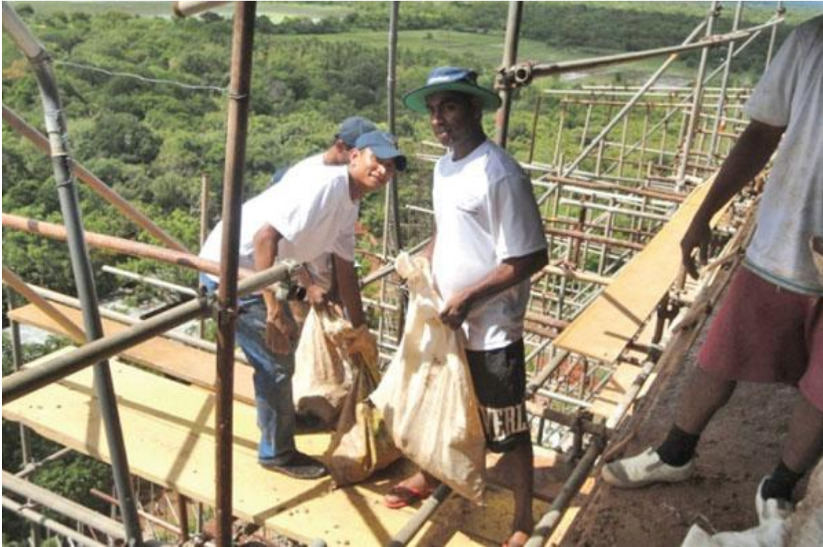
Hauling stones for the restoration
