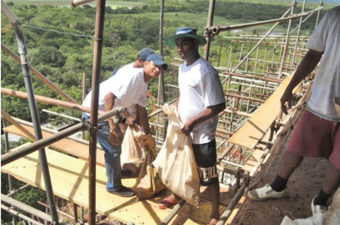
Hauling stones for the restoration
