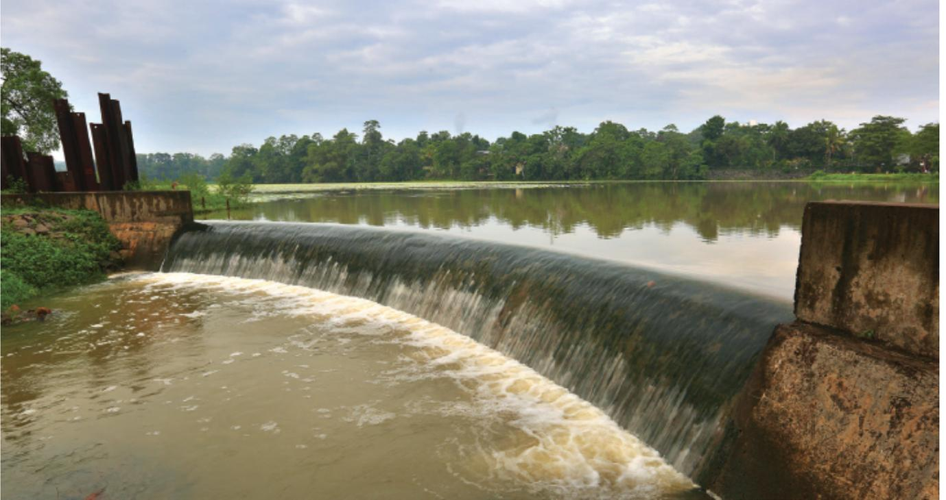
The spillway removes excess water from the tank, while adding to its charm.
