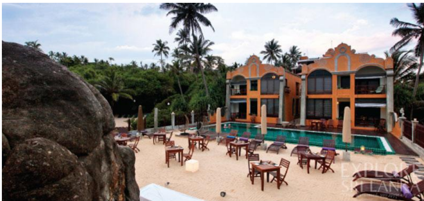
The rear view of the Resort
