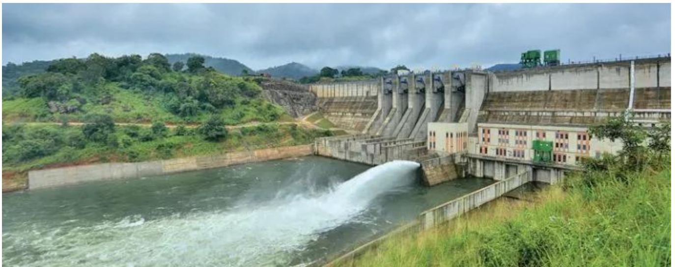
The hydro electricity power station at the base of the dam
