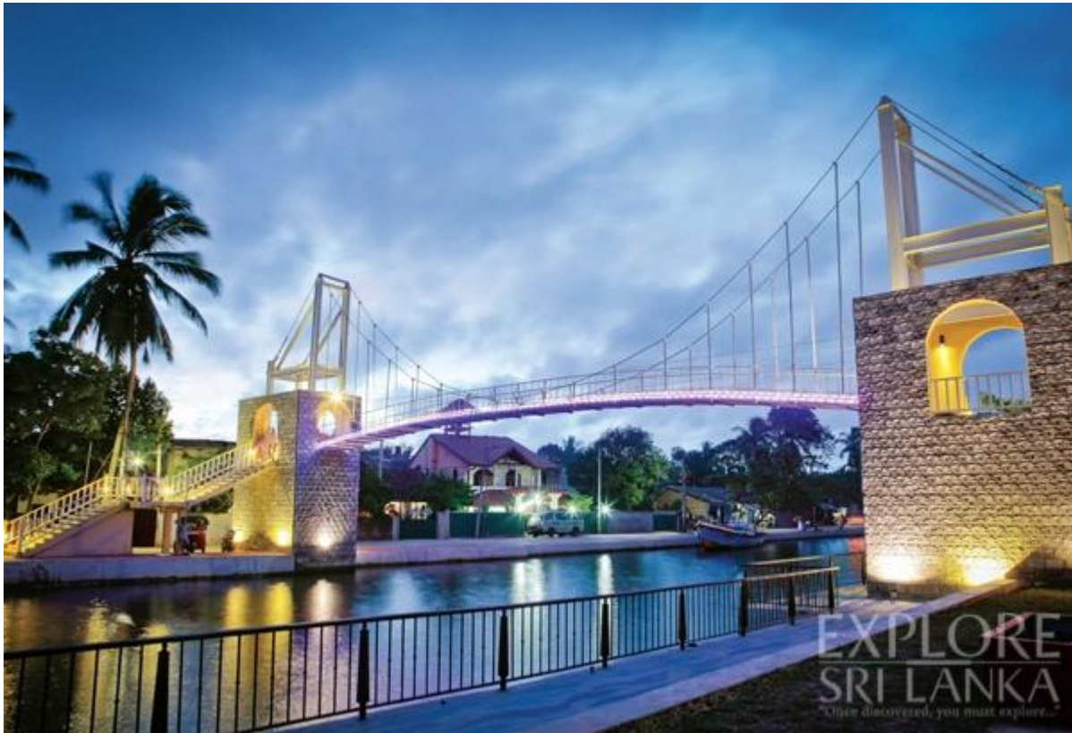
The new suspension bridge for pedestrians
