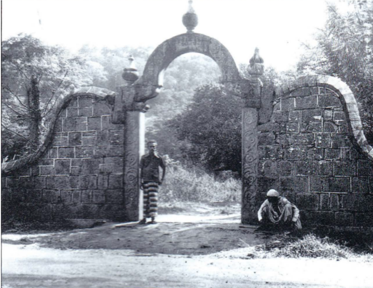
The stone arch gateway to the Black Prince's home.
