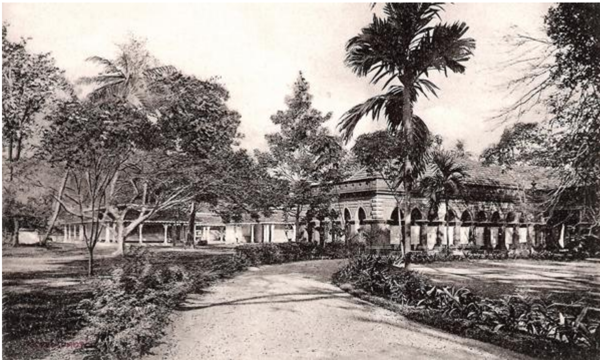
The Lady Havelock Hospital c. 1910 (Photograph: Skeen & Co)
