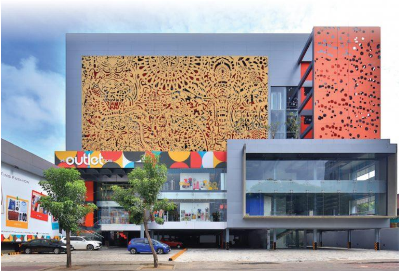
The striking façade of the store
