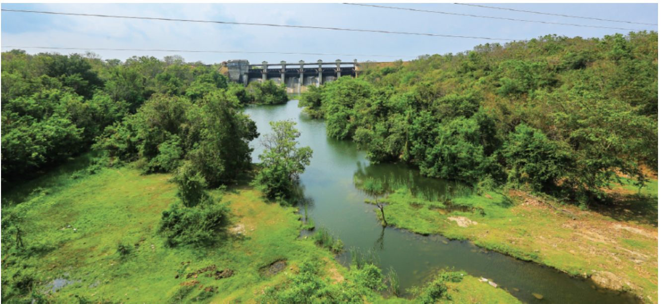
The impressive structure of the sluice gates of the Lunugamvehera reservoir.
