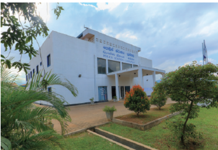
The Police Station is an eco-friendly space.
