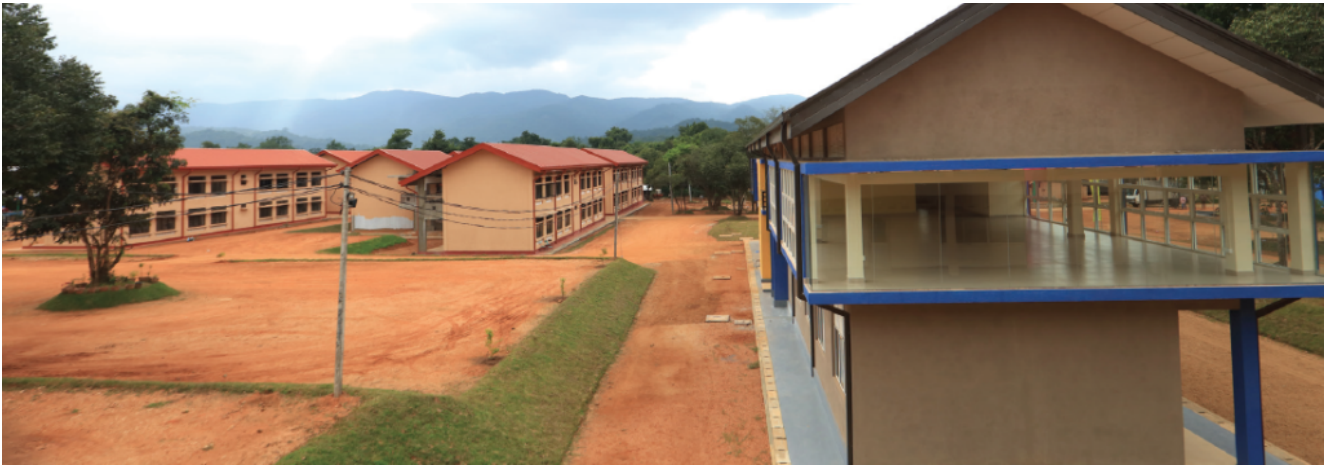
The Pallegama Central College is one of the five schools built in the Laggala Green Town.
