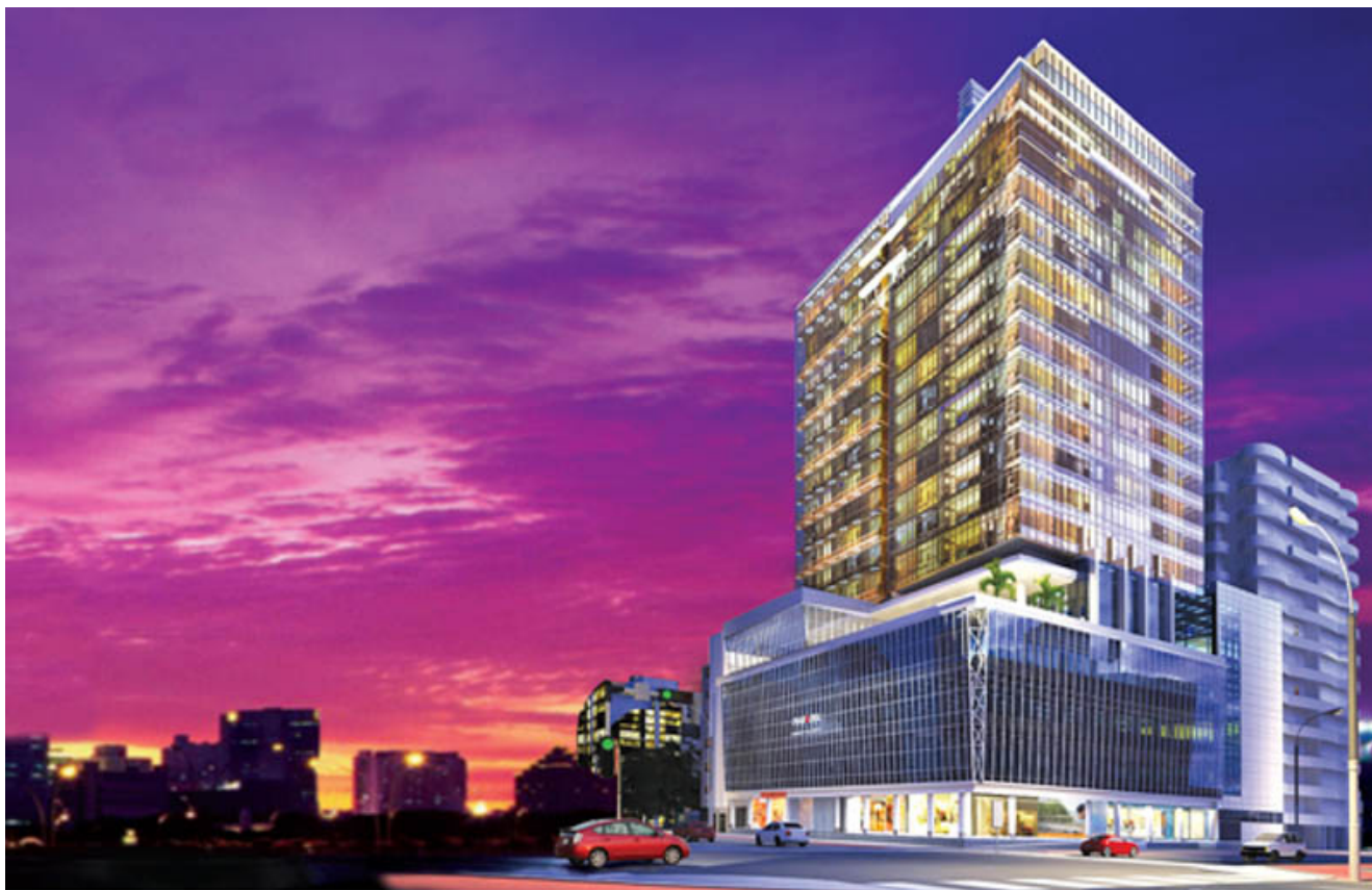
Exterior of Platinum 1 once completed
