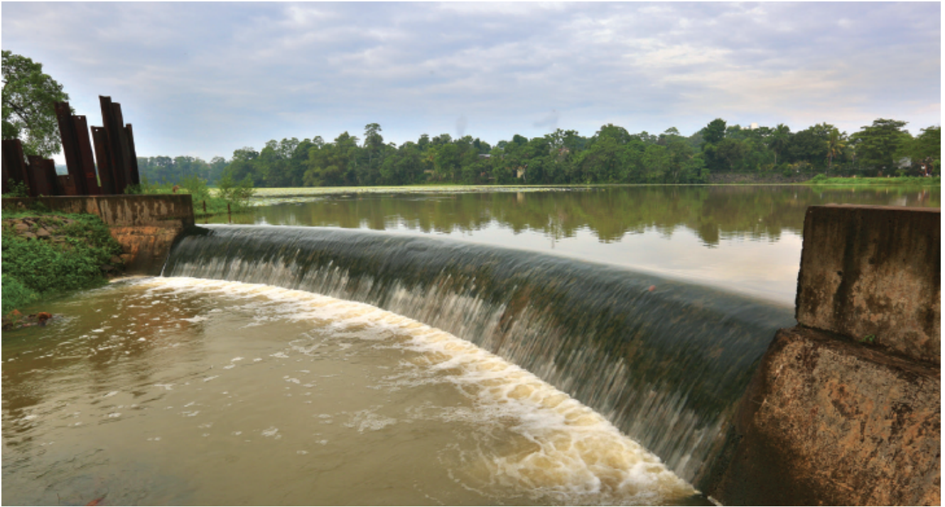
The spillway removes excess water from the tank, while adding to its charm.
