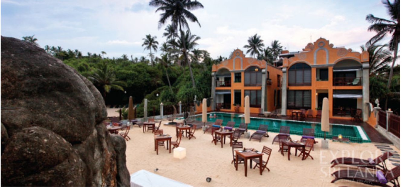
The rear view of the Resort
